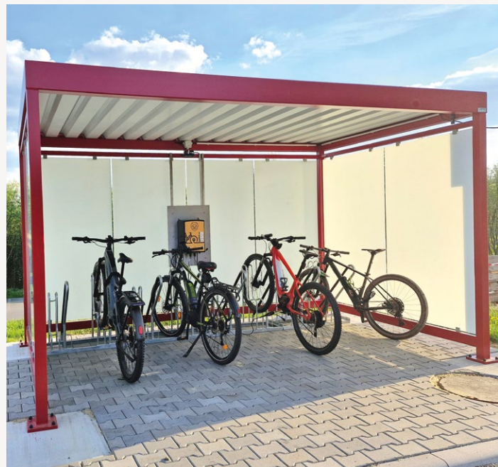
Bicycle shelter with charging station for e-bikes
